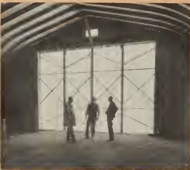
GEORGE DUFFY, UNITED FARMERS' PRE-CUTTING PLANT MANAGER; LAWRENCE STONE; CLIFF FAULKNER, ASSOCIATE EDITOR OF THE COUNTRY GUIDE; PICTURED IN MR. STONE'S ARCH RIB BUILDING WHICH FEATURES THE TRANSLUCENT FILON-FACED DOOR.
