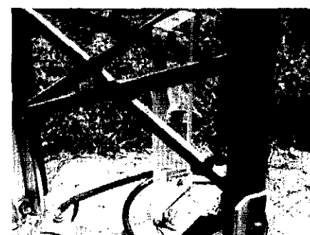
A plastic block mounted on a right-angle bracket at the tower base serves to support an antenna loading coil.
