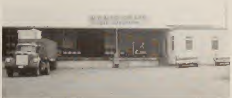
Petroleum Warehouse with the office shown at the right.
